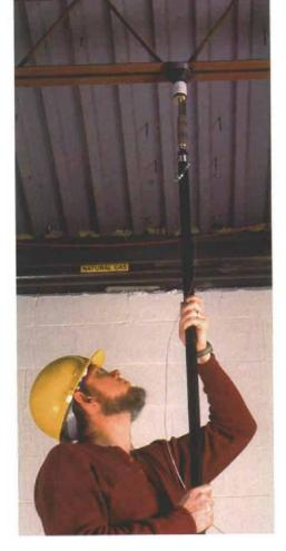
**No more climbing on ladders.** ITW Ramset's single-shot L1600 LADD tool shoots preassembled pin-and-clip assemblies into concrete or steel for tying off suspended-ceiling grids.
